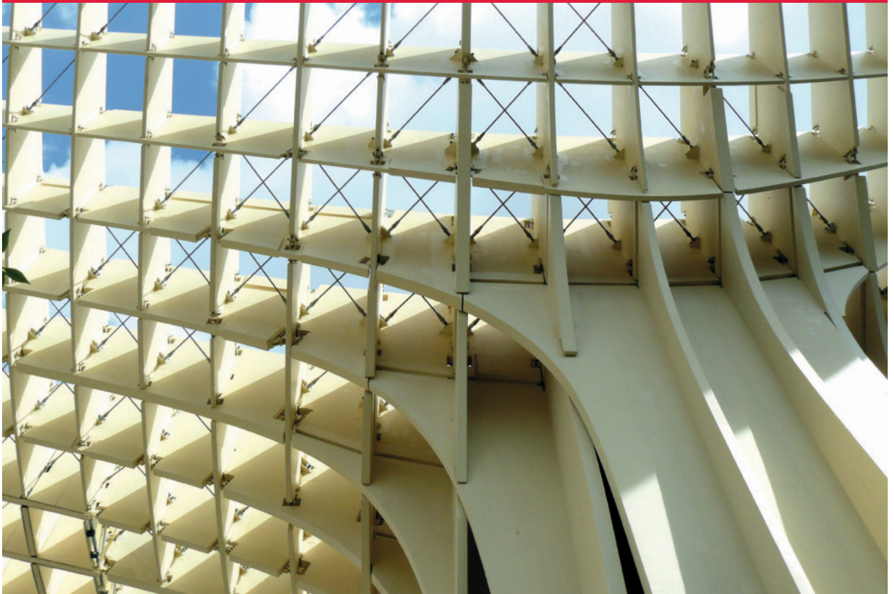
High-tech construction in wood: Parasols over the "Plaza de la Incernacion" in Seville
