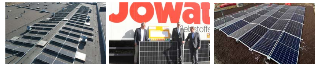
We rely on renewable energies, e.g. from solar panels on roofs like pictured here in Poland, Malaysia, Switzerland and Detmold.
